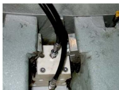
BEKAWIND retrofit kit contains all fastening elements, hoses (filled with grease) and fittings.
